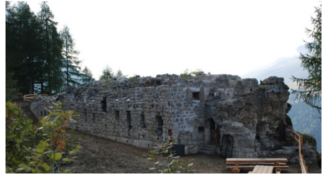
Fig. 13 - Forte Pozzi Alti ( http://www.trentinograndeguerra.it/context.jsp?area=100&ID_LINK=242&id_context=149 [23/08/2019]).
